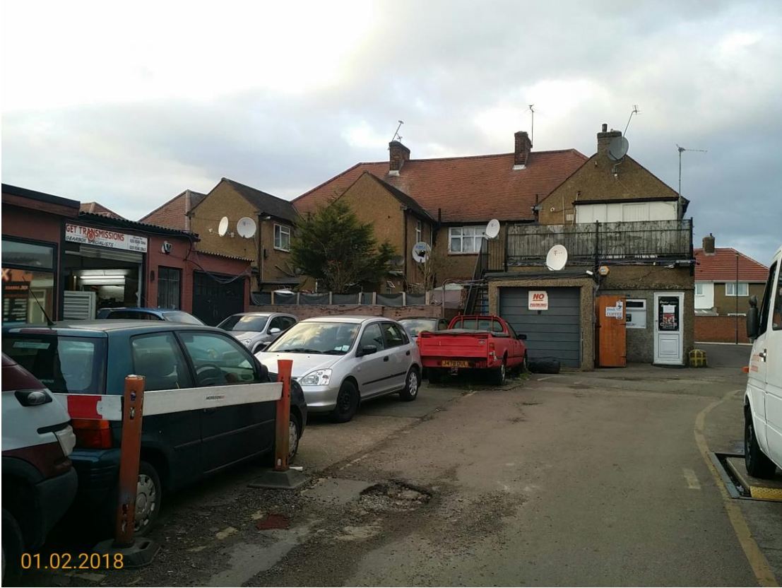
Rear of properties on Bacon Lane
