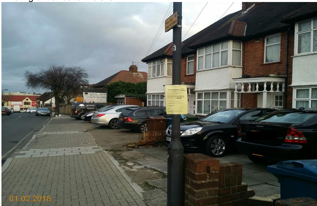
Properties 1 -5 Bacon Lane to be demolished
